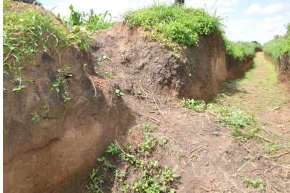
Figure 3. A spot in QEPA where elephants destroyed a bank of a trench to cross from the park to a cultivated field
